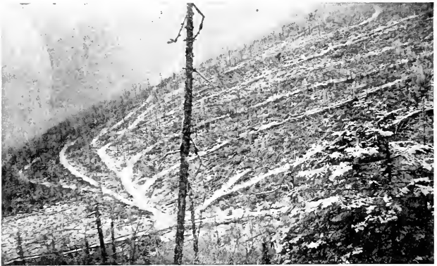
FIG. 42. — Yarding-sled Trails leading down to a Skidway on a Two-sled Road. Maine.
